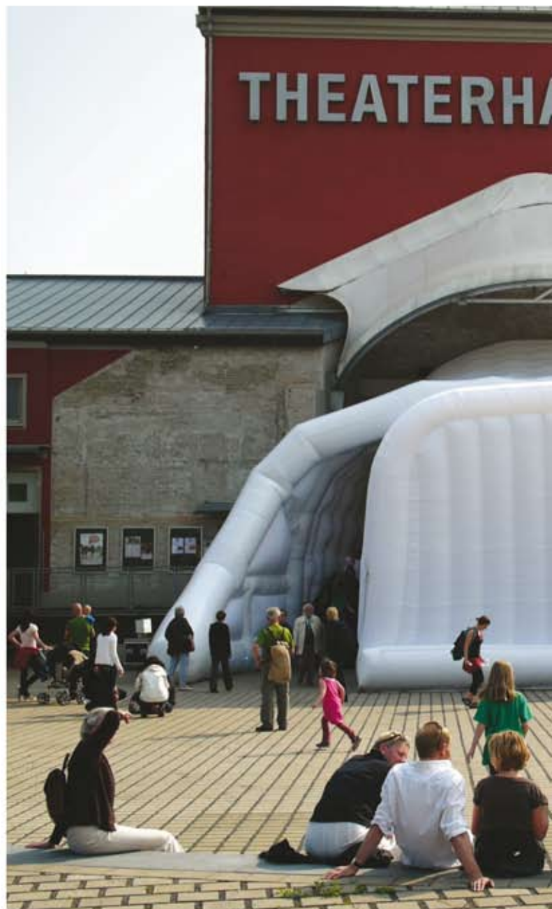
The extension, made from 3,000sq m of PVC-coated polyester weave, is prepared for its inflation.
